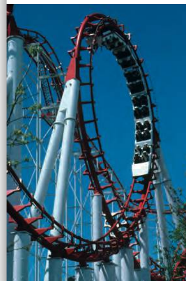
If the ride is propelled by gravity then the designer must make sure that the car has this minimum speed when it reaches the top.
