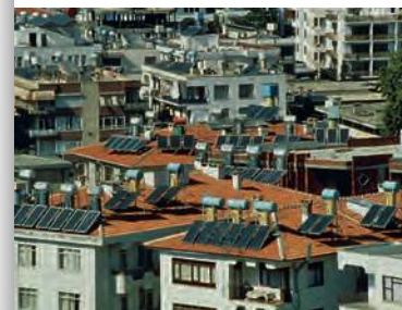
Solar heating panels on top of houses in Antalya. The position of solar panels depends on the amount and direction of sunlight as well as the design of the building and other considerations.
